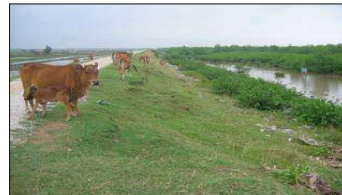
5km seadyke at Thai Do with mangroves protection was totally safe after the same storm
