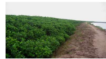
Unconcrete seadyke in Giao Thuy
