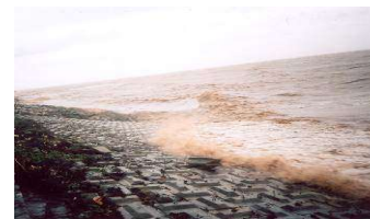
Concrete sea dyke in Do Son, Hai Phong
