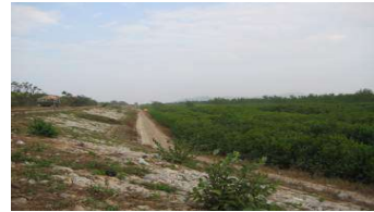
The sea dyke in Bang La was protected with mangroves
